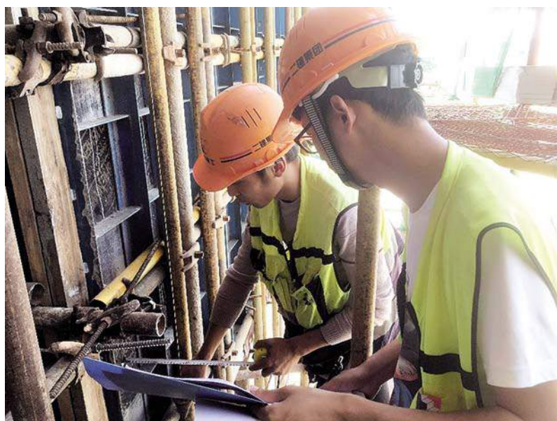
墙柱模板垂直度自检
